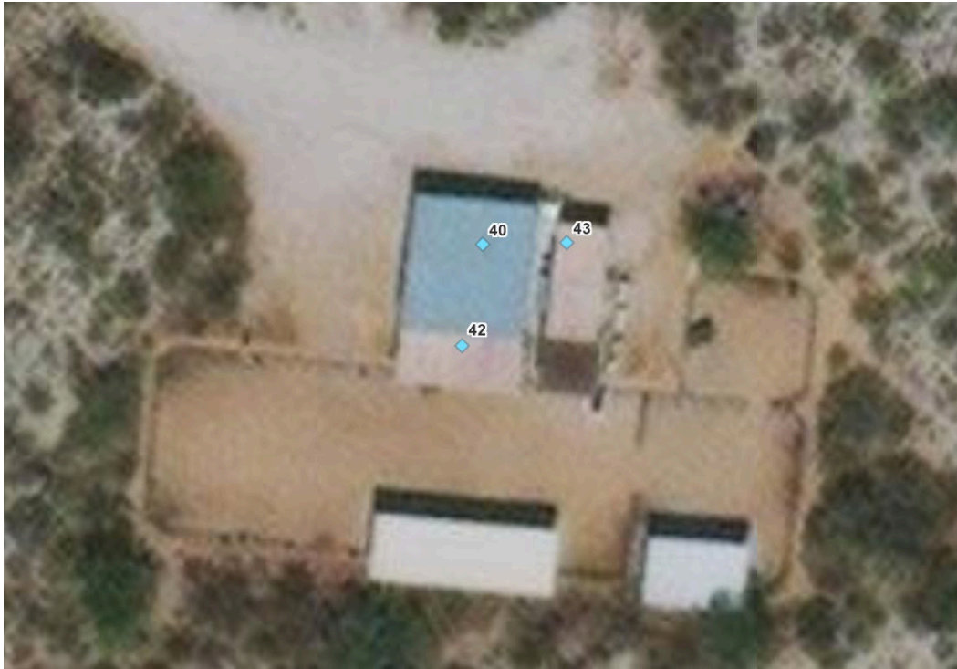
Figure 20. Specified Retrofits for the Horse Corral
