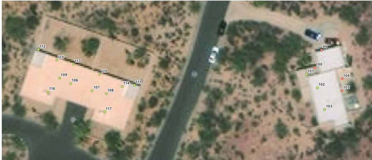
Figure 13. Fixture Compliance with Dark Sky Guidelines for Quarters 30, 31, and 32. Dark sky compliant lighting has a green marker and non-compliant lighting has a red marker.
